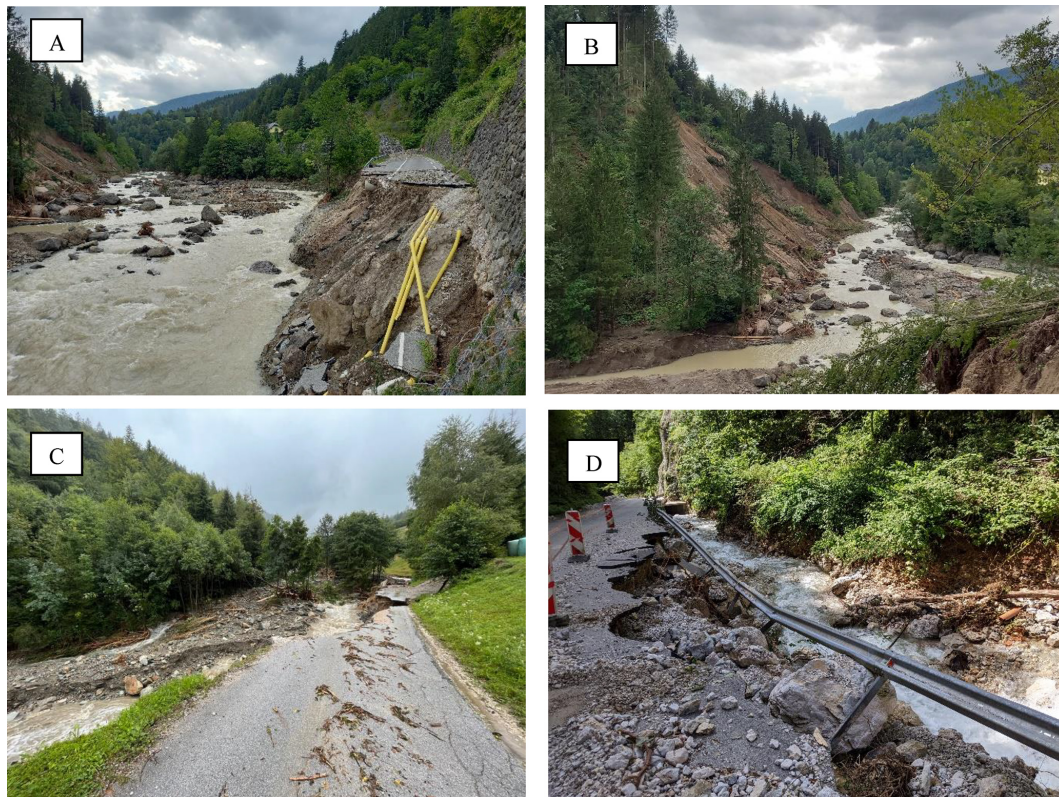
Figure 4. Photographs of bank erosion and infrastructure damage (panels a , c and d ) and mass movement processes (landslide in panel b ) across Slovenia during the extreme August 2023 floods, with focus on the upper Savinja River catchment (some photographs courtesy of Igor Benko).
