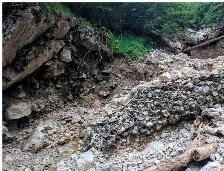
**Figure 5.** One example of the consequences of the May 2018 event on the existing infrastructure in both torrents: a partially destroyed already filled flexible barrier.
