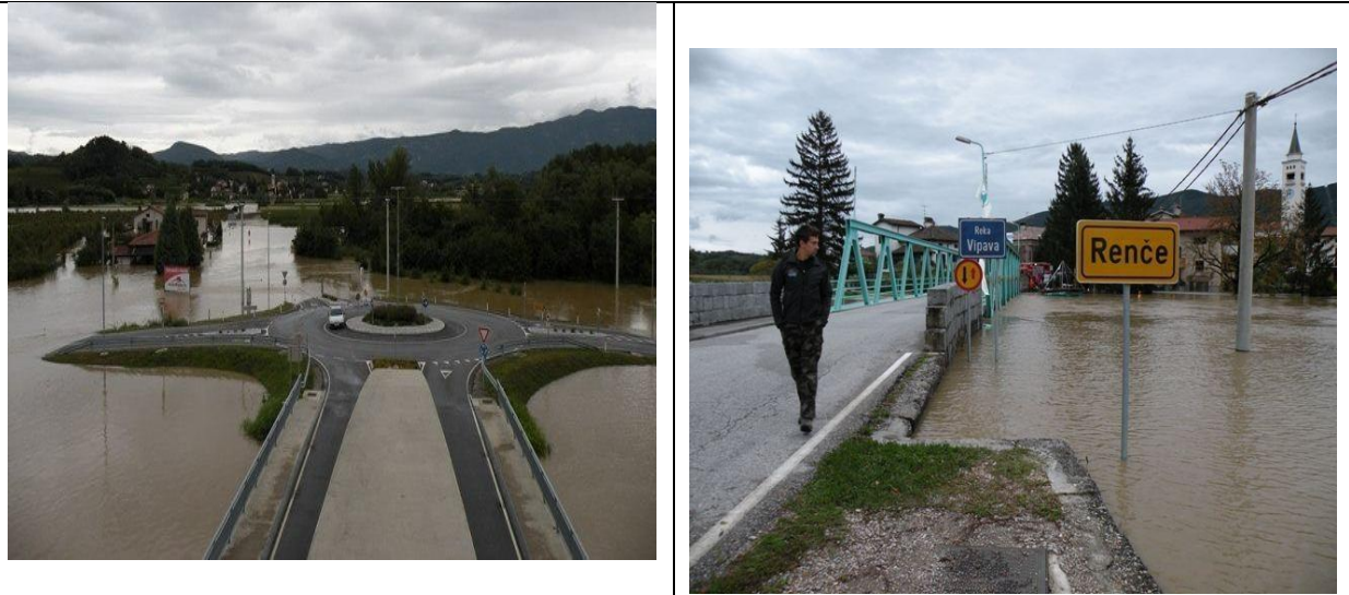
Figure 3: In September 2010, a flood reached the bridge deck, and many streets were closed due to the flooding.
