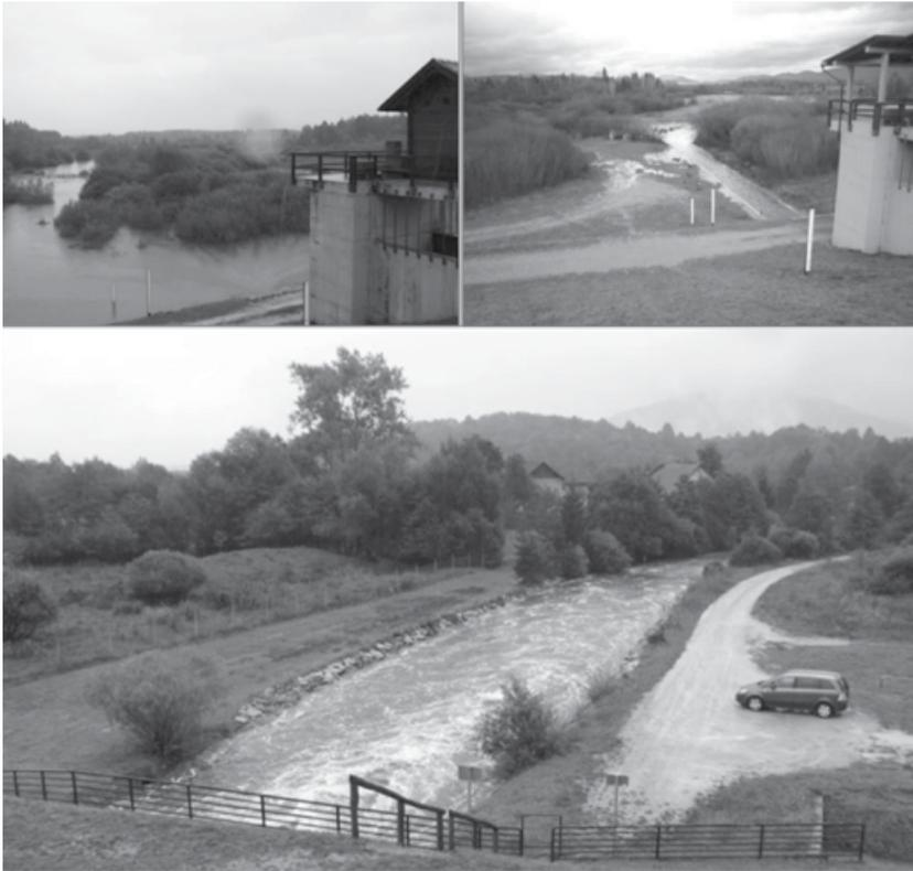
Notes: Upper two photos show the area inside the retention reservoir during high- (left) and low- (right) flow conditions. The lower image shows reservoir outlet flow during a high-flow event.
