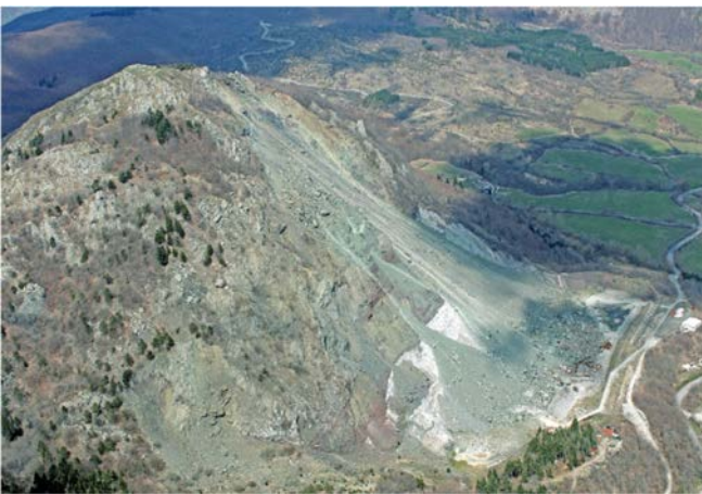
Fig. 9 Second place—Impact of the Monte Beni rockslide on both the regional roadway SR 65 and the quarrying activity—by William Frodella (Department of Earth Sciences, University of Florence, Italy)
